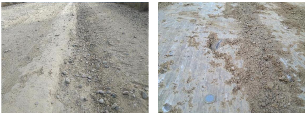
Figure 22.11. Original surface (left) and surface after gravel removing (right).
