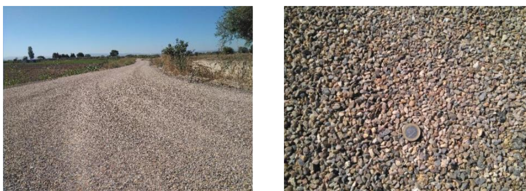
Figure 22.15. Bituminous surface dressing(S-EST3).
