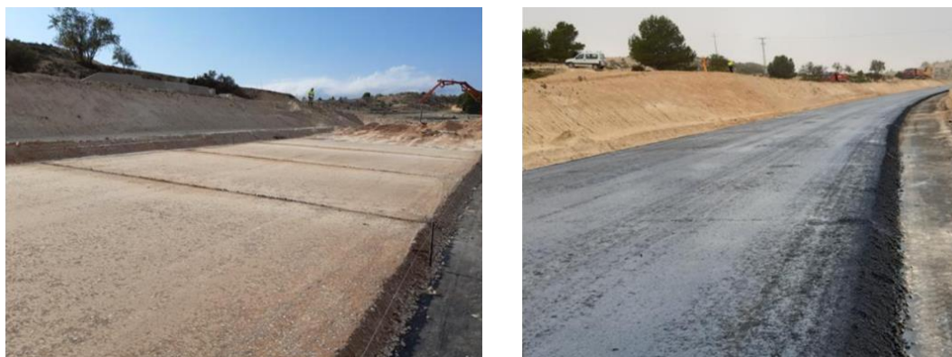
Figure 22.18. Appearance of pre-cracking layer and soil-cement cover with curing emulsion.
