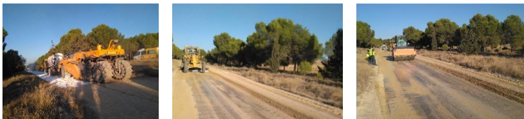
Figure 22.12. Soil stabilization process: 3% WPFA dosing and mixing, levelling and compacting.
