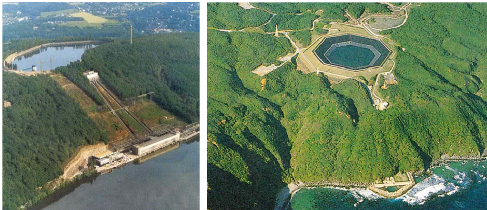
Figure 3.3 Images corresponding to two different PHES installations.
