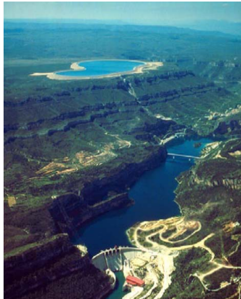
Figure 3.4 Cortes- La Muela PHEs facility complex in València, Spain.
