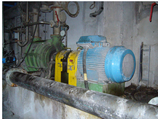
Figure 4.7 Vacuum pump in a paper mill
