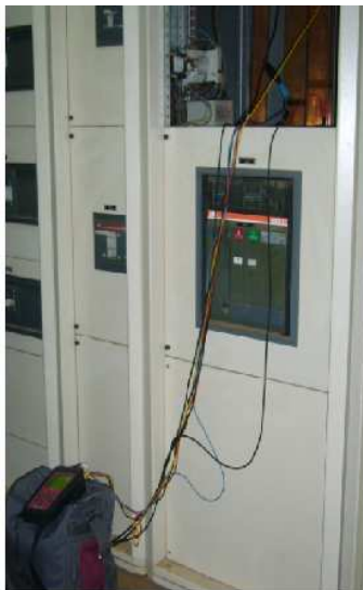
Figure 5.7 Power system analyser - Portable. Circutor AR5. Switched in a general bus-bars of a plant.
