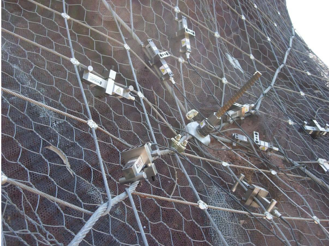
Figure 7.- Sensors set up in Carmona. Typical arrangement.
