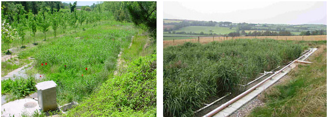
Figure 1. A) Horizontal Sub-Surface Flow Constructed Wetland located in Les Franqueses del Vallés, Catalonia (Spain) ( www.ingeniabios.com ). B) Picture of a vertical subsurface flow reed bed constructed wetland in Ireland ( www.wasteworks.ie ).
