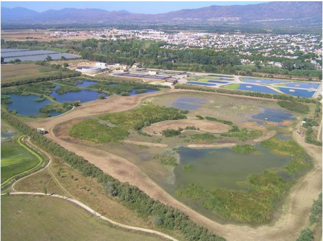
Figure 9. The Empuriabrava Wastewater Treatment Plant and adjacent FWS constructed wetland. Photograph: Ll. Sala.
