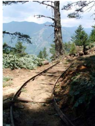
Figure-1.8.- Rehabilitation of the abandoned mining railway
