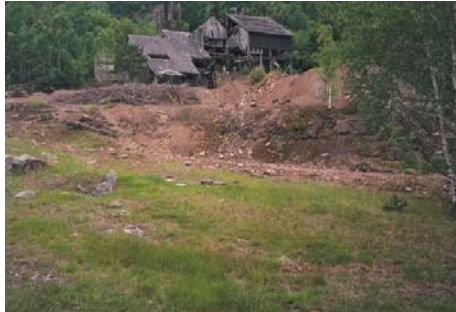
Figure-1.5.- View of Pontaut treatment factory
