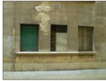
Figure III.45: The repeated appearance of fenced windows in C/del Baluart, Barceloneta, Barcelona (Spain): territorial intensification
